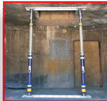
Ceiling & Wall Shoring
